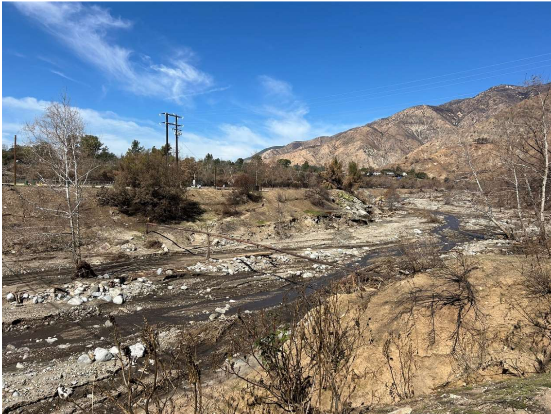
Photo looking NW at pipe crossing Eaton Wash following the February 14, 2025 Debris Flow
